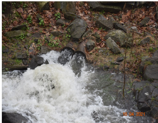
Fig. 4: Small valves opened during the controlled release.
