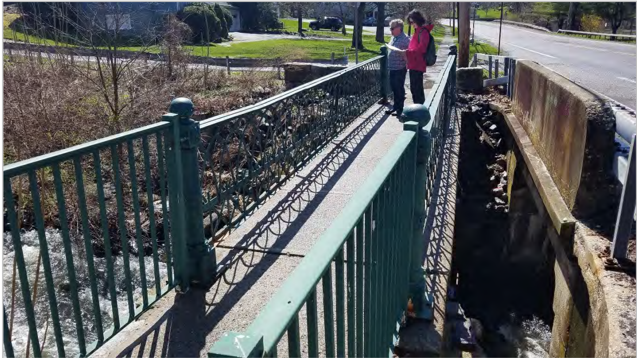
Landsman Kill historic pedestrian bridge
