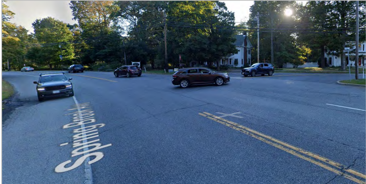
Wide intersection at Route 9/Springbrook/Montgomery; drivers using the shoulder to bypass left turning-vehicles (source: Google maps; image capture: 2019)
