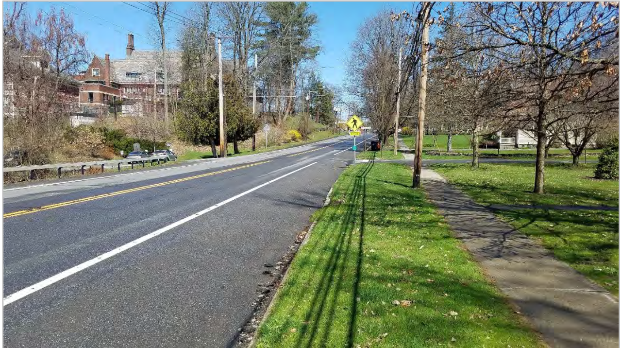
Route 9 looking northbound towards Legion Park entrance; note wide shoulder and sidewalk buffer
