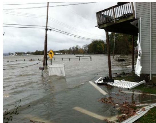
View of flooded road in Stony Point following Hurricane Sandy in 2012 (L. Konopko)
