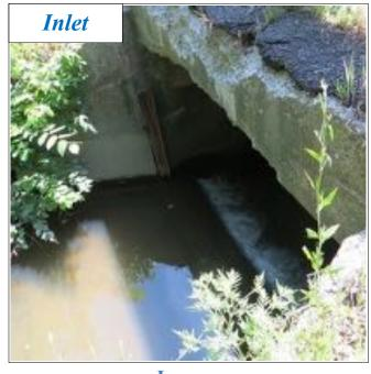
Inlet Shape/Type: Wingwalls Inlet Drop/Grade: Inlet Drop Width: 10 Height: 7
